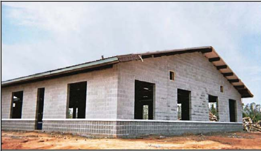
6000 blocks including numerous window openings and cast concrete sills complete in 4 days.
