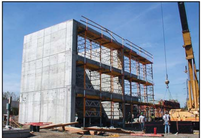
Construction of the specialty manufacturing facility required both damage limiting interior walls and explosion venting exterior walls.
