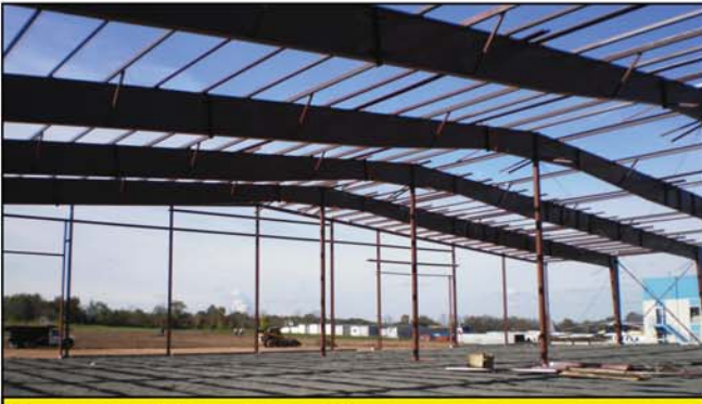
Erection of steel for warehouse addition
