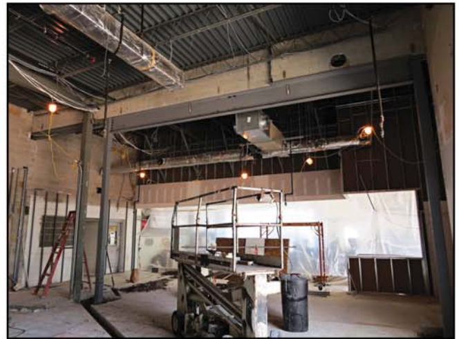
Newly installed support beam
