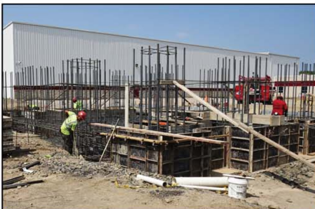
Piers prepped and ready to receive concrete
