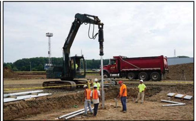
Beginning of helical pile installation
