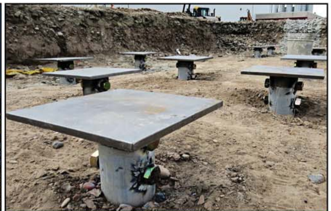
Cut and capped helical piles
