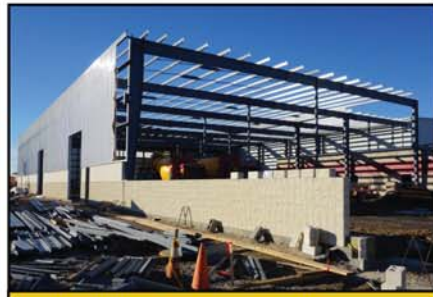
Steel installation nearing completion
