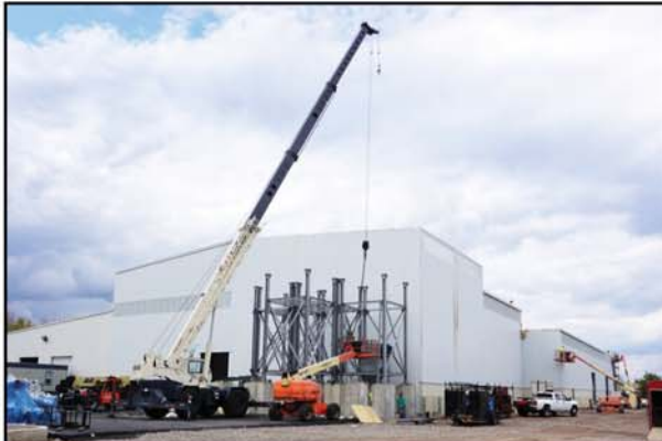
Installation of silo supports
