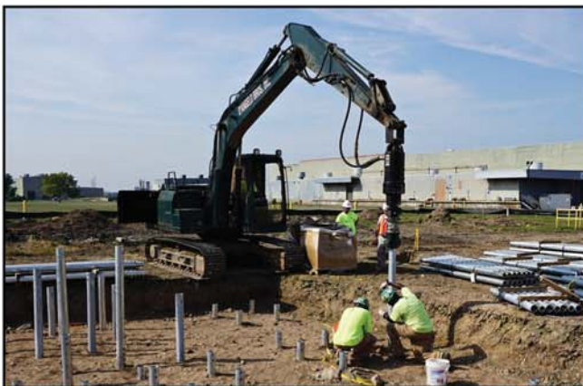
Helical pile installation continues.
