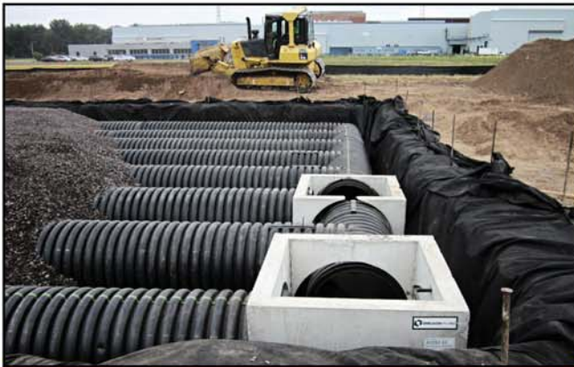
Underground storm water basin
