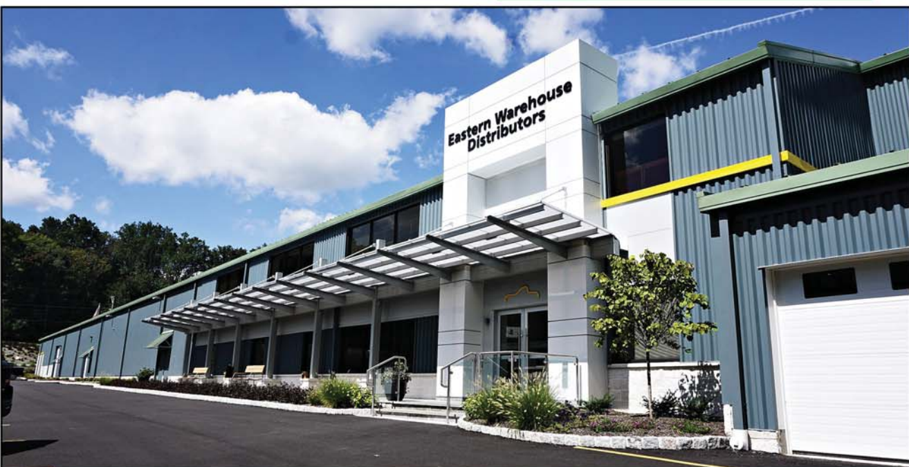
ACM clad tower at main entrance
