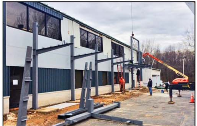
Installation of the reverse angle canopy
