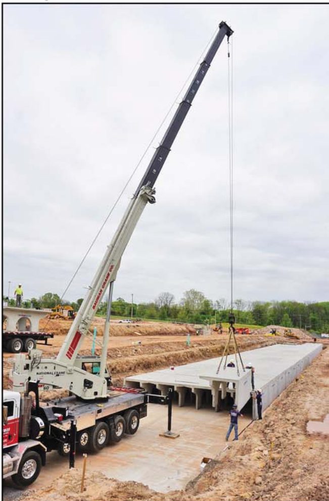
Installation of Underground Detention Basin Structure
