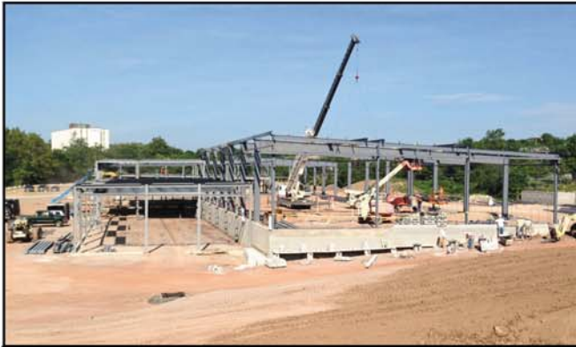
Structural Steel Erection
