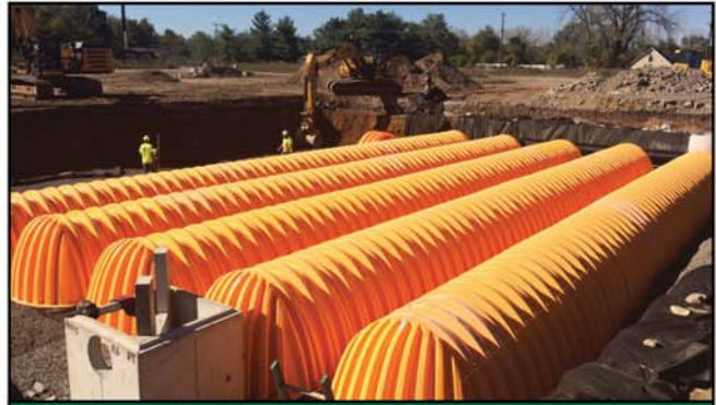
Installation of StormTech Chambers
