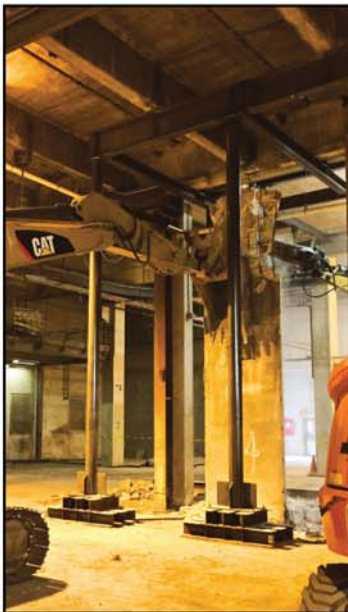
Support Steel for Wall Removal
