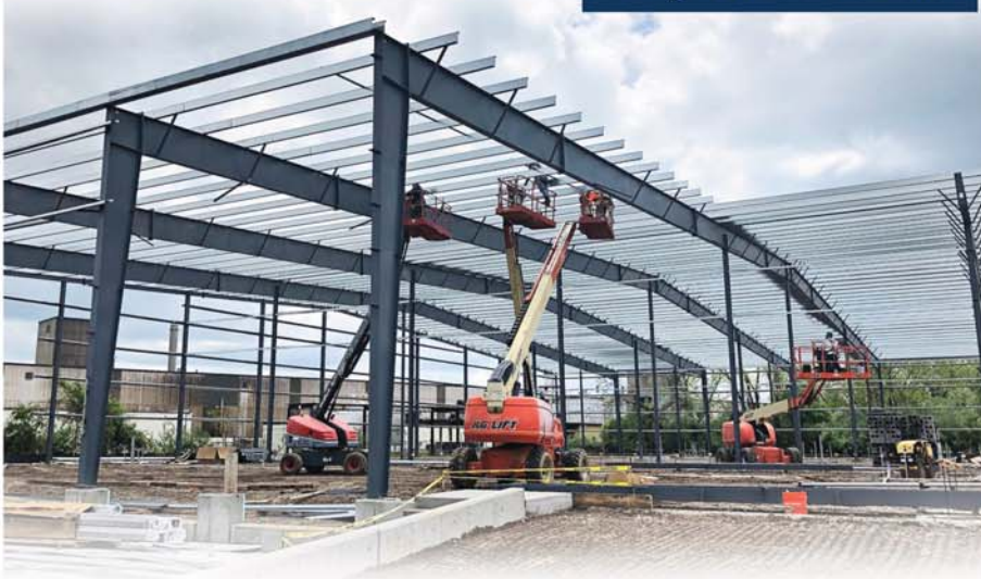
Pre-engineered steel installation
