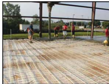
Installation of radiant heat system at Barrett
